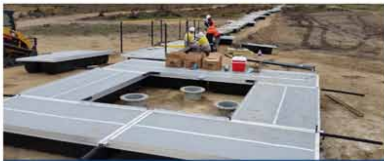
500m being Installed in Kwazulu Natal South Africa
